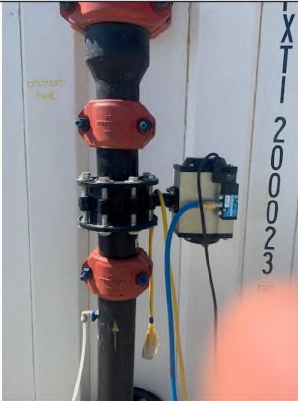
Automatic Shut Off Valve Set Up: Functioning with Automatic Shut-off
