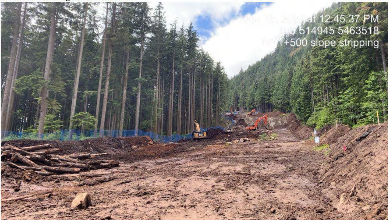
Photo 3: Stripping at the KP 1+500 slope. Water management with the installation of cross drains on the ROW has improved overall site drainage at this location.
